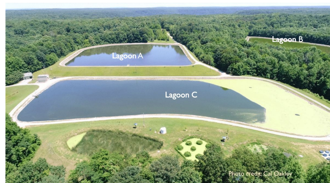
Figure 1A Aerial View of lagoons Algae assimilate excess nitrogen and decompose. Depth allows for denitrification of organic nitrogen.
