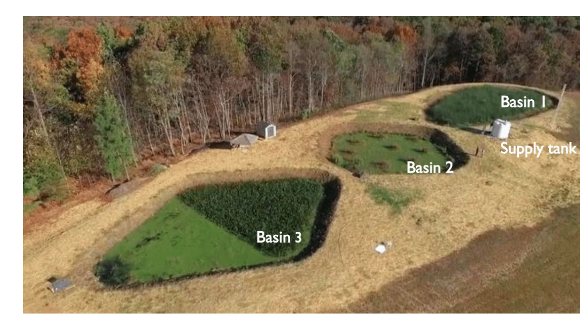
Figure 1C Aerial view of constructed wetland basins. Wetland utilizes algae and plant assimilation and photosynthetic zones as tertiary treatment.
