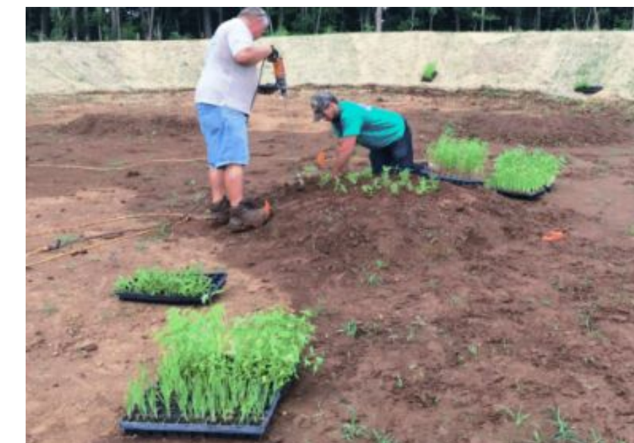
Figure 1B Planting of vegetation during wetland construction designed to assimilate ammonia.
